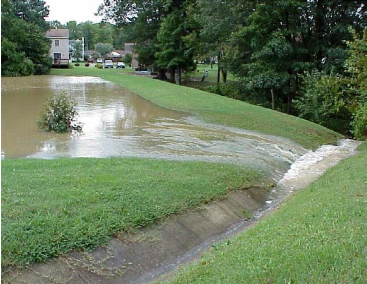
*Figure C-2. Emergency Spillway Draining into a Concrete Channel*
