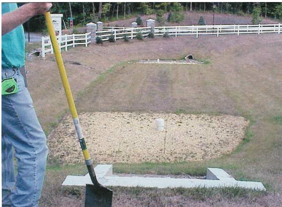
Figure 12.3. Hybrid Sand filter in a Detention Basin
