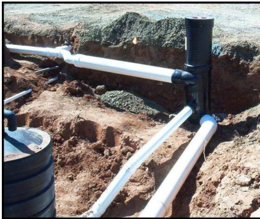
Figure 6.11. Installation of Vortex Filter prior to backfill
