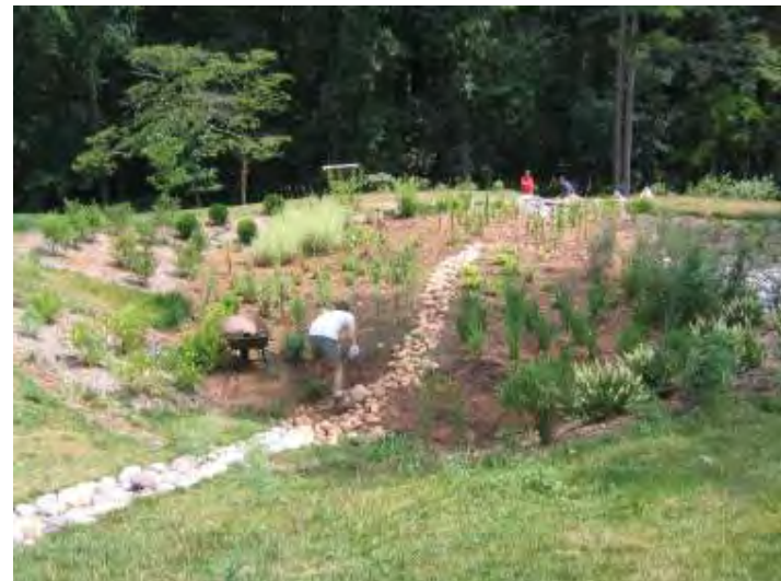
Install plant materials and water until established
