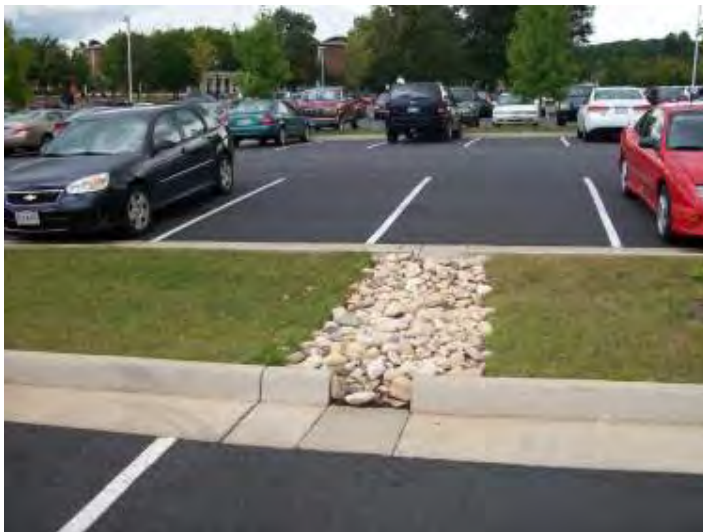
Stone too high at inlet – blocks flow
