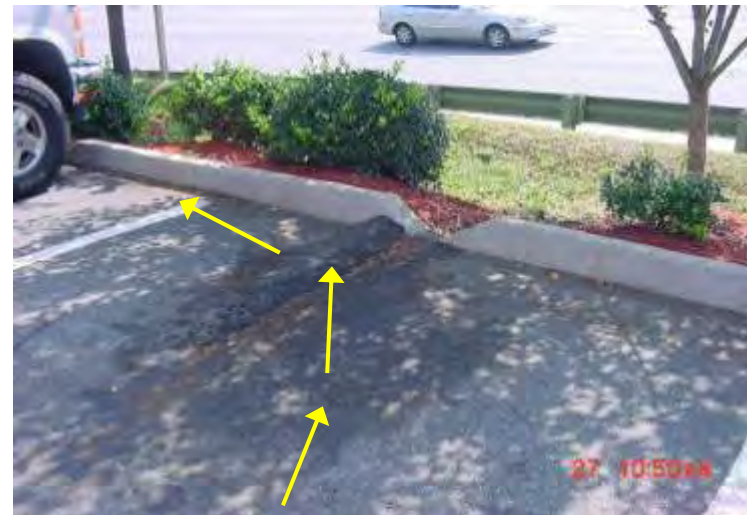
Small grade changes divert flow from inlet
