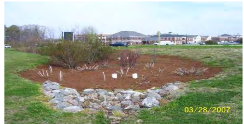
Stone/Rip Rap Apron
