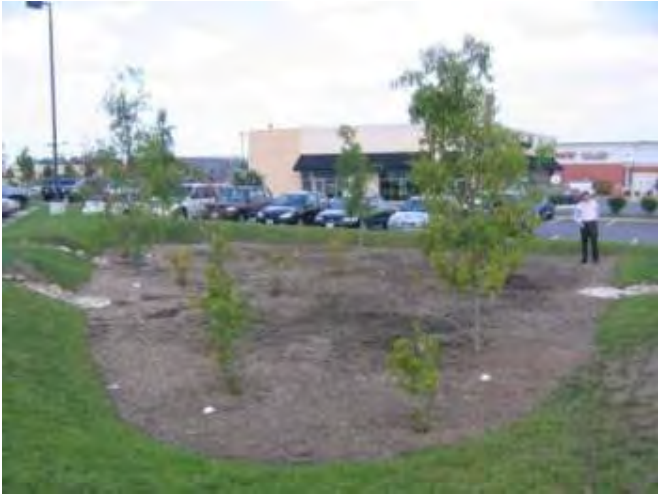
Parking Lot Edges
