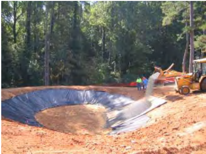
Install geotextile on SIDES ONLY (optional), add gravel to create stone storage layer up to design elevation
