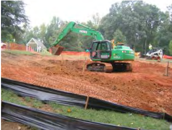
Install secondary E&S, excavate from side
