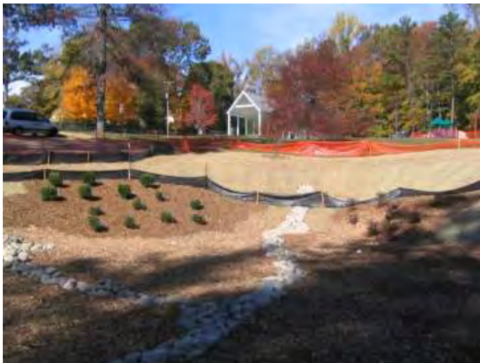
Install surface cover: mulch, stone, matting, etc.
