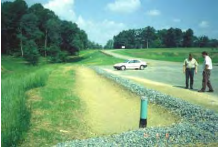
Installed too early during construction
