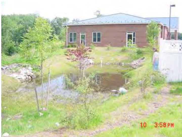
Sediment clogs filter surface
