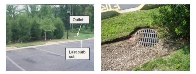
Figure 9.11. Examples of Short-Circuiting at Bioretention Facilities
