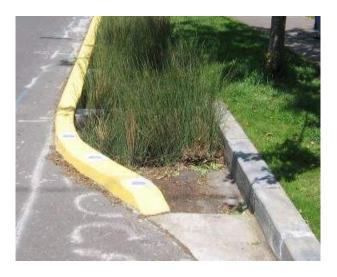
Figure 9-A.3. Stormwater Curb Extensions
