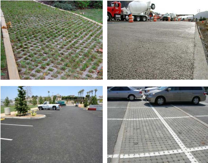
**Figure 7.1. Types of Permeable Pavement:** (clockwise from upper left): **Concrete Grid Pavers** (Chesapeake Stormwater Network); **Pervious Concrete** ([www.pervious.pavement.org](http://www.pervious.pavement.org)), **Porous Asphalt** (UC Davis) **Permeable Interlocking Concrete Pavers** (UC Davis)
